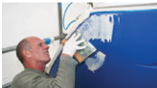
Fairing any defects
