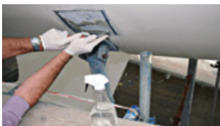
Wet scrape to remove old antifouling
