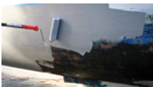
Apply Underwater Primer onto prepared surface
