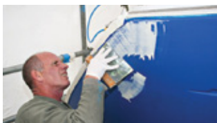
Fairing any defects
